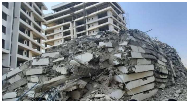
Figure 3. Scene of 1 November 2021 Ikoyi building collapse (The Guardian 2021b).
