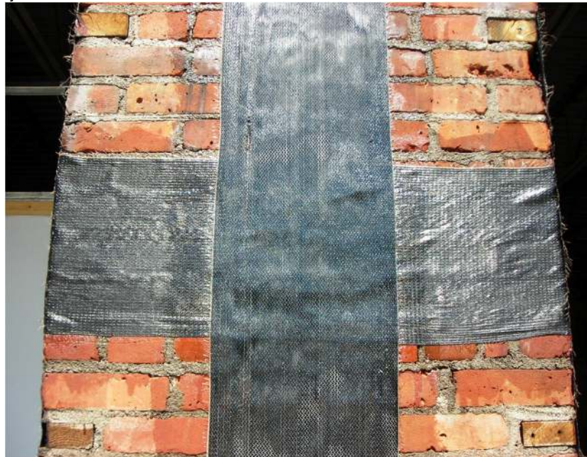
Figure 2.5: Unidirectional carbon fibre strips on masonry (Houlette, 2011).
