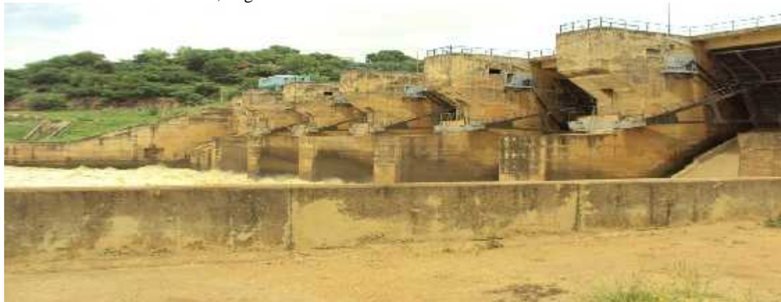
Fig. 1a: Side view of the dam wall
