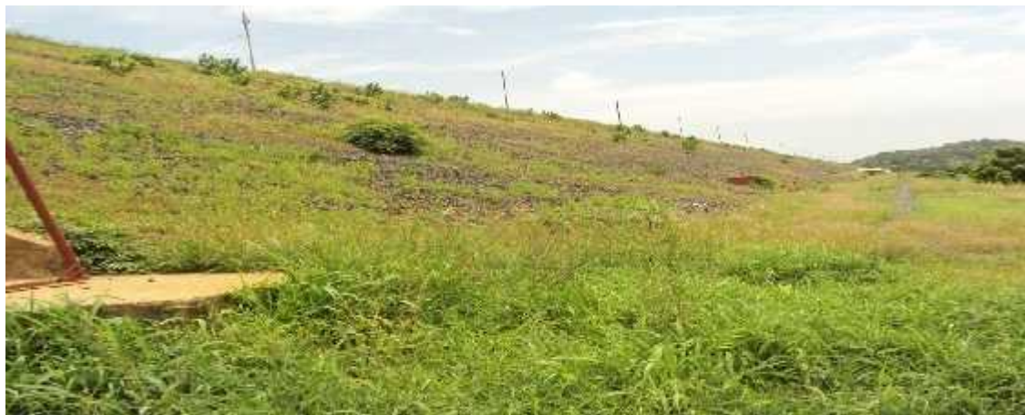
Fig. 1b: Extension of the dam wall
