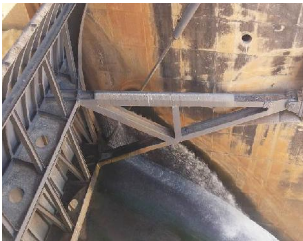
Figure 2: (a) leakage at the wicket gate (b) leakage at the pump house
