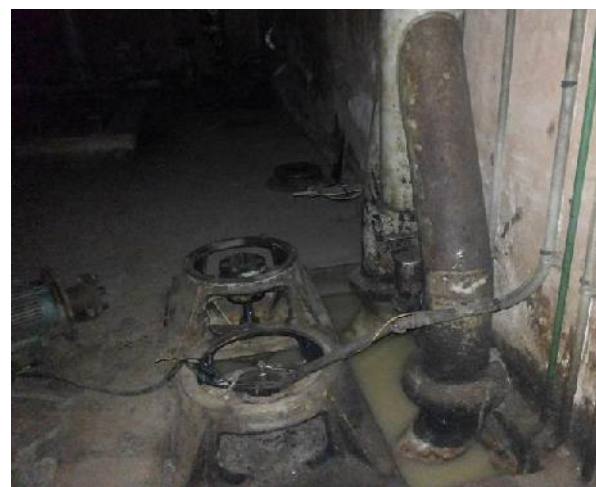
Figure 2: (a) leakage at the wicket gate (b) leakage at the pump house
